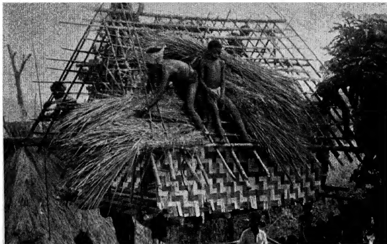
Thatching the roof of a field house.
